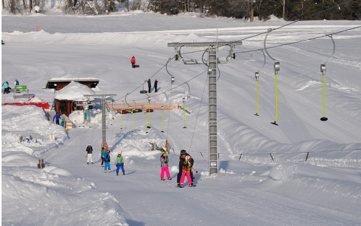
Straight supports, large cable sheave, high cable – the LUIS LIFT surprises with its details.
